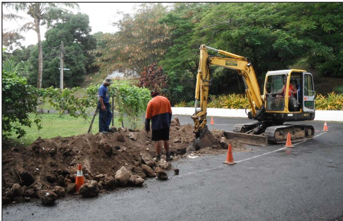
Connecting cross mains at Victoria Rd & Ara Metua
